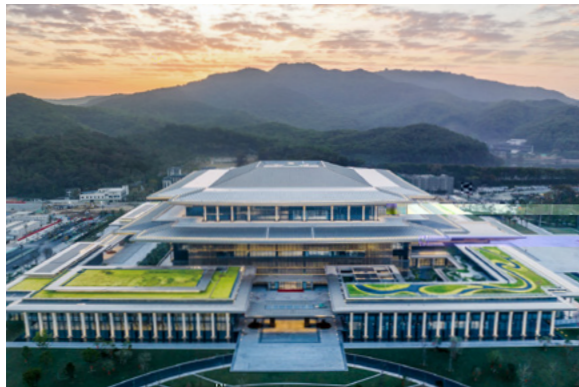
Baiyun International Conference Center Phase II
